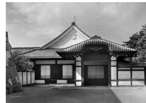
Nagoya Castle's restored Honmaru Palace and its entrance and carriage porch before they were burned down during the war
