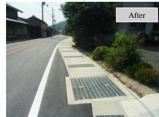
Gratings were installed on a street with a narrow sidewalk
