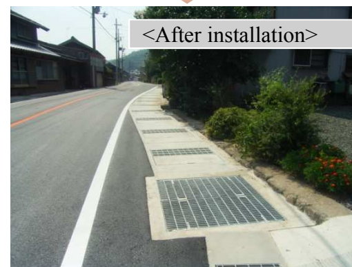
Gratings were installed on a street with little sidewalk width
