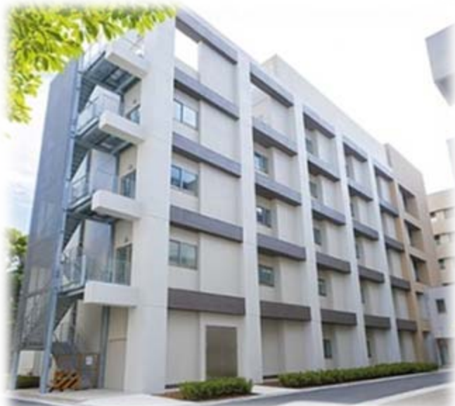
New research building of the Advanced Medical Research Center of Yokohama City University
