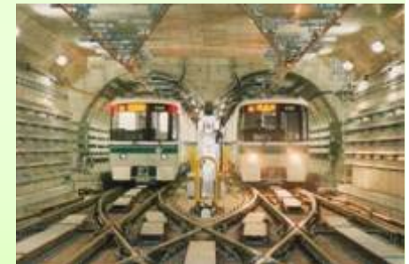
Municipal Subway Kaigan-line (Yumekamome)
