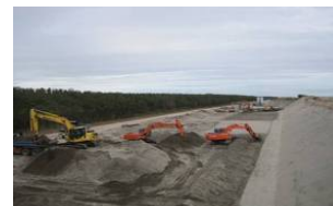
浜松市沿岸の防潮堤
