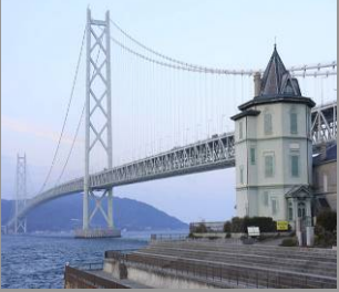
① Akashi Kaikyo Bridge
